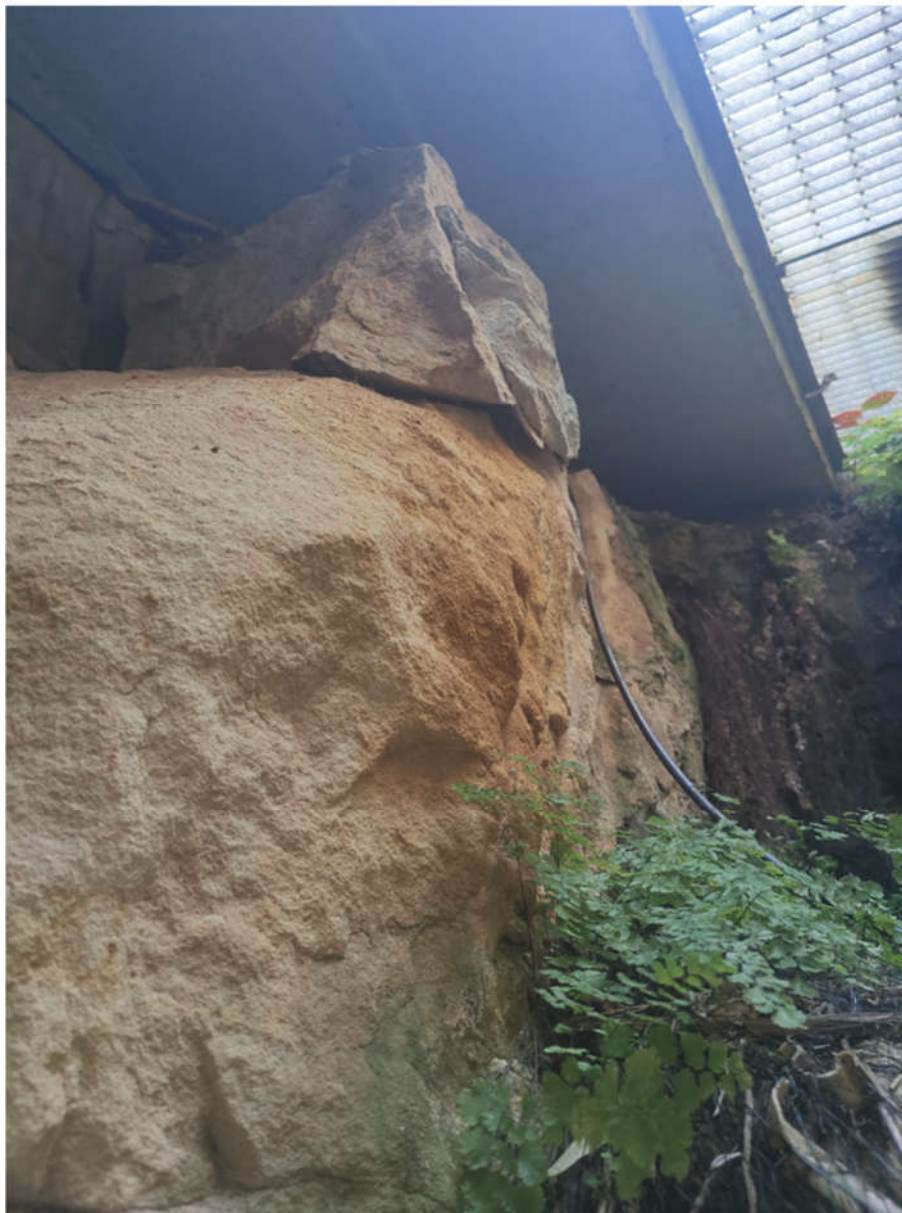
Plate 1a - Block of Rock (Boulder size) at Crest of Sandstone Cutting (Southern Boundary)
